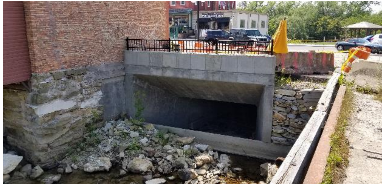
Center Street Overflow Culvert
